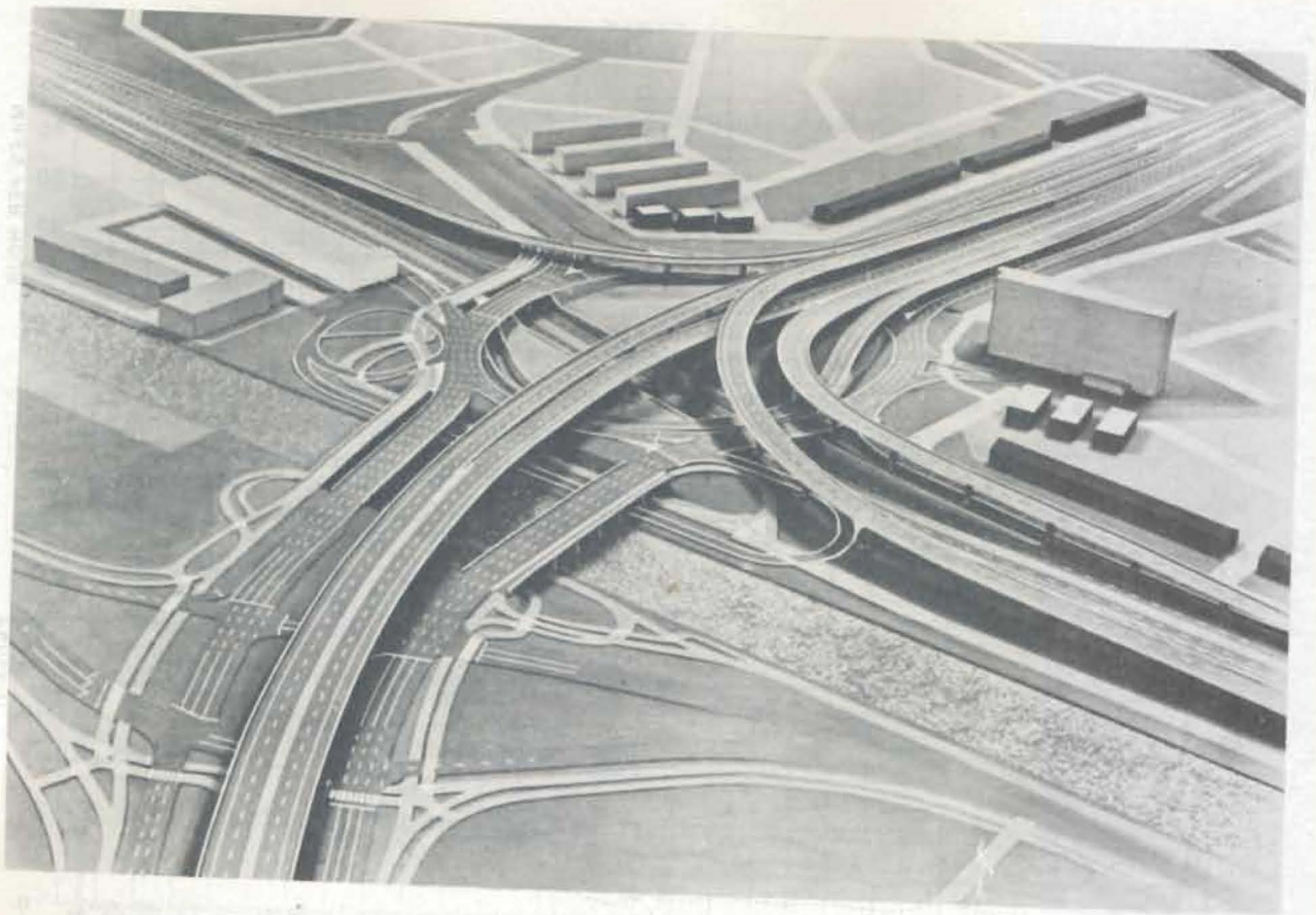
Figure 3 - Model of Interchange North of Rotterdam, Netherlands
