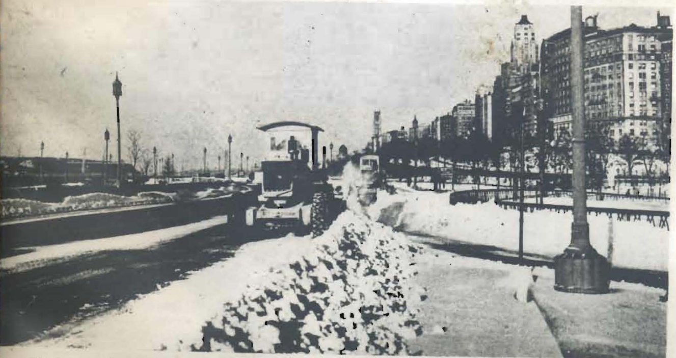
Fig. 1.—Snow Broom Mounted on Caterpillar Motor Grader, Operating on the West Side Express Highway
